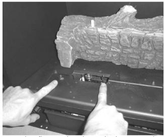
The left log has two holes in the bottom that fit over the pin on the burner and metal bracket attached to the pilot assembly.
